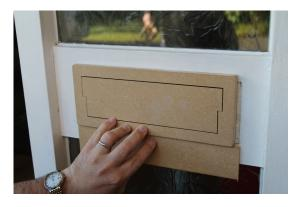
Holding the Letterplate Eco in place, fix the fitting bar to the door with masking tape. This provides a guide line for fitting and will support the Letterplate Eco as the sealant sets.
