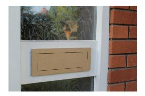
Once your Letterplate Eco is fitted and the sealant has cured, remove the fitting bar and all tape. Touch up parts of the letterbox surround as needed for a neat finish.
