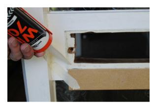
Apply a thin bead of silicone sealant on the door around the flat front edge of the aperture.
