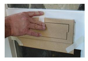
Once cured the sealant will support and keep the Letterplate Eco in place without the tape.
