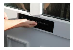
Still without sealant, put the Letterplate Eco into the aperture with the flap pushed completely to the top of the unit and as far up in the hole in your door as it will go, ie you can't push the whole unit any higher in the aperture with the flap held open.
